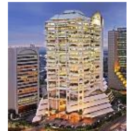
Intiland Tower Jakarta
